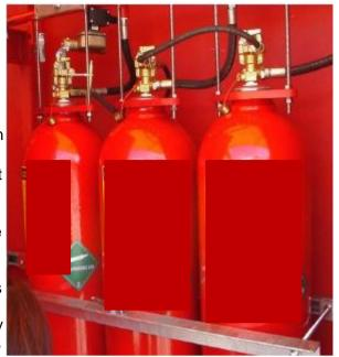
The K85 Valve c/w Cylinder is factory filled with carbon dioxide. A single cylinder may be used, or multiple cylinders can be manifold together to obtain the required quantity of agent for total flooding or local application methods. The K85 valve can be actuated electrically, pneumatically, and / or manually with the appropriate valve actuation components.
